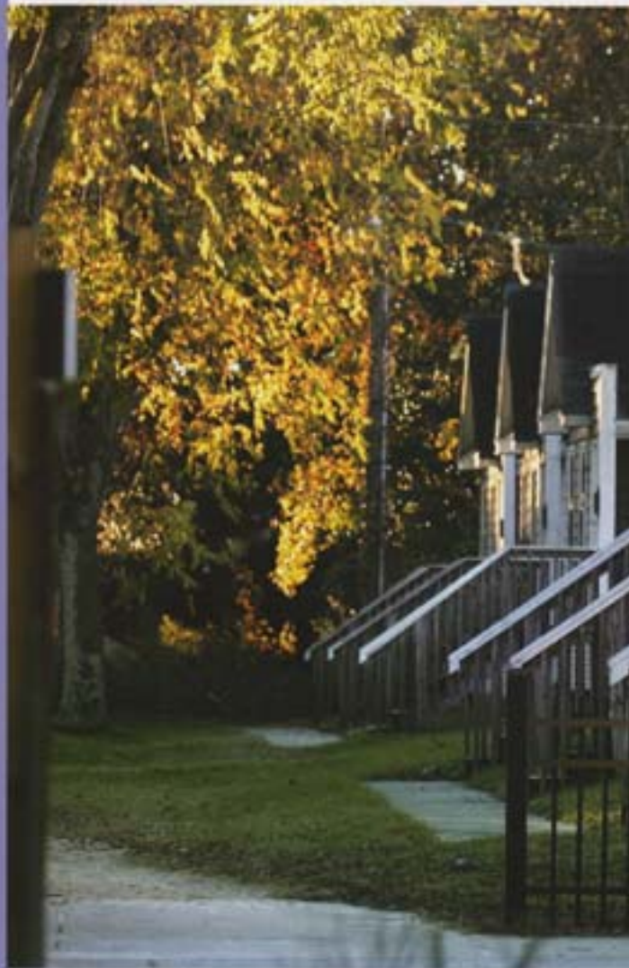
These Charleston Cottages provide transitional housing for formerly homeless persons. The design won an Honor Award from the American Institute of Architects.
